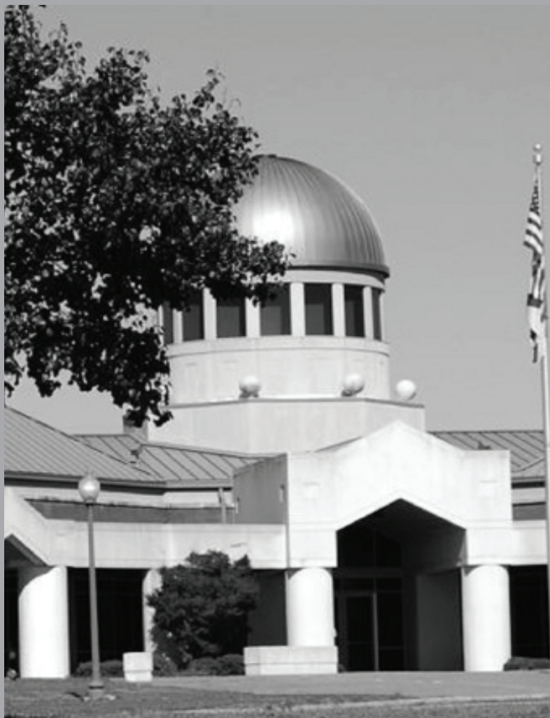
Administration Building, Opelika Campus
