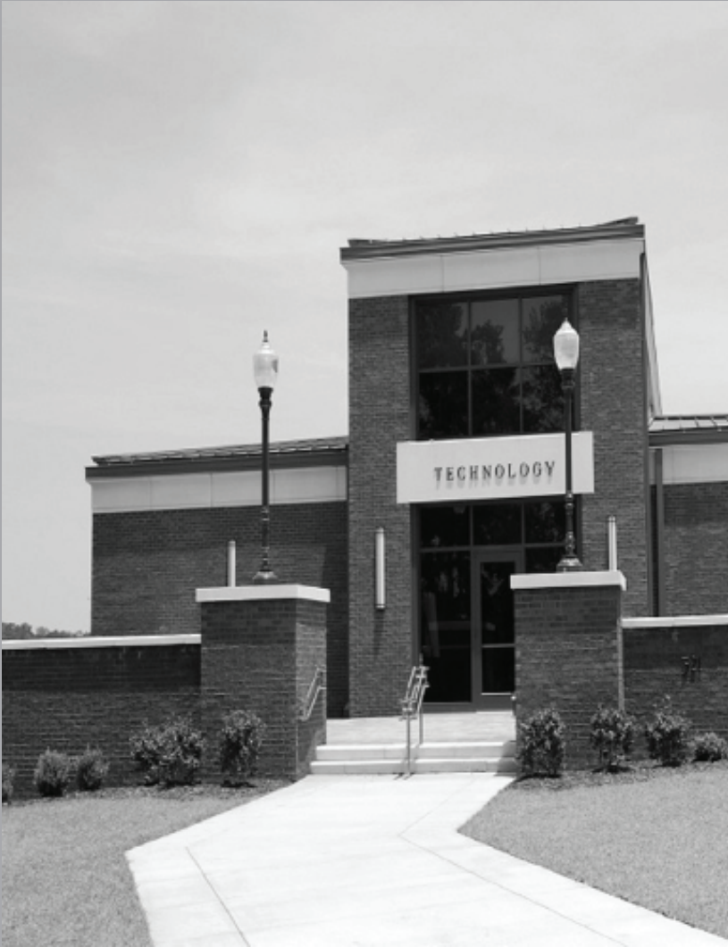
Technology Building, Valley Campus
