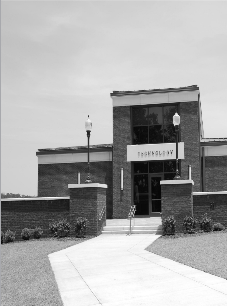
Technology Building, Valley Campus
