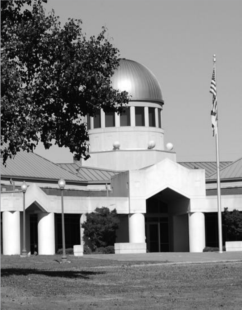
Administration Building, Opelika Campus
